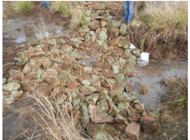
Rocks being used to slow the flow
